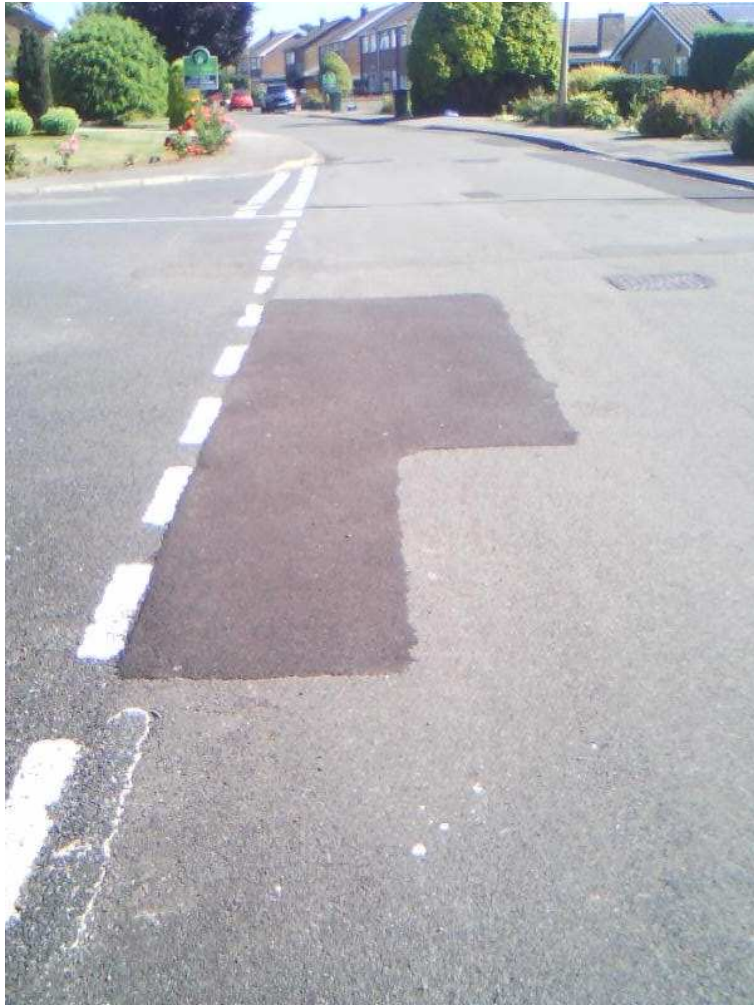
This shows the P5 patch has not deteriorated during the winter season.
